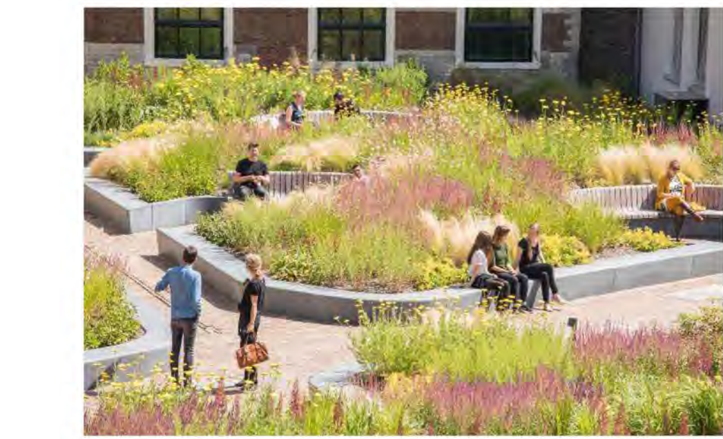
RAISED PLANTER WALLS @ COURTYARD: CONCRETE, POUR-IN-PLACE, NATURAL GRAY (NO COLOR)
