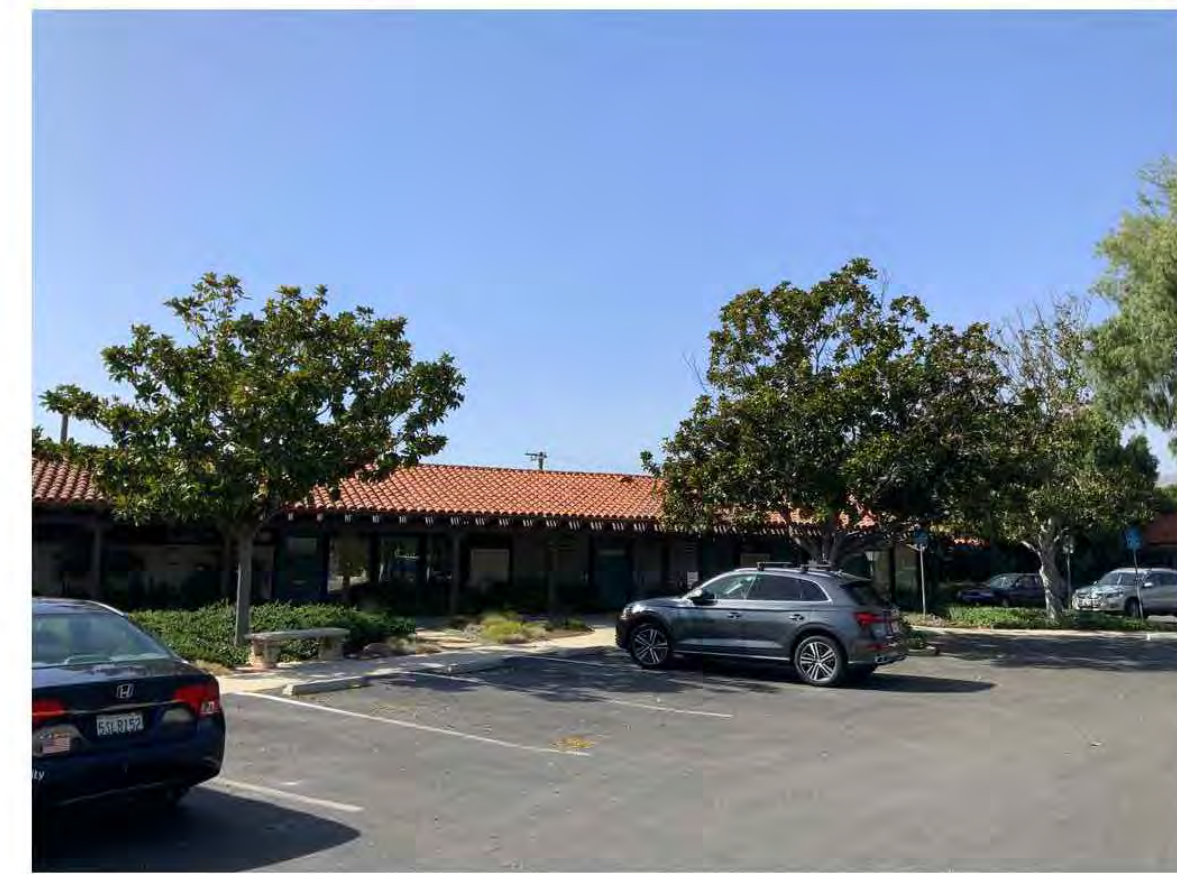
Above: Another perspective of Mags and euc interior to site, to be removed. Below: South side of bldg. Carrotwood trees along Via Lucero to be removed.
